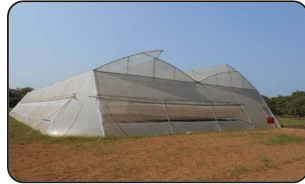
Polyhouse constructed under RKVY
